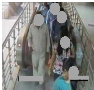
Figure 1 Escalator in operation at a Delhi metro station
